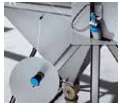
Level monitoring in the dust hopper
